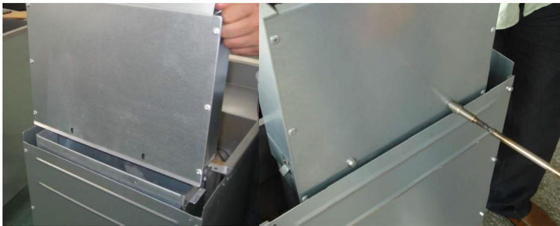
3. Slide the flue wrap over the flue.      4. Secure it with four self-tapping screws, two on the back and one on each side using a 5/16" socket.
