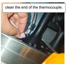
• If the trouble still occurs,, Remove the thermocouple connector at the gas valve end again, light the pilot, and continuously press the knob to ignite for more than 10 seconds. Measure the thermoelectric voltage of thermocouples, it must be greater than 24mv, otherwise the thermocouple needs to be replaced.
